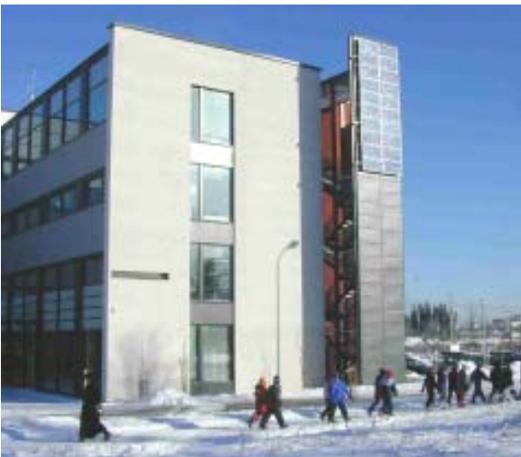
Modules retrofitted as cladding elements over the wall.
