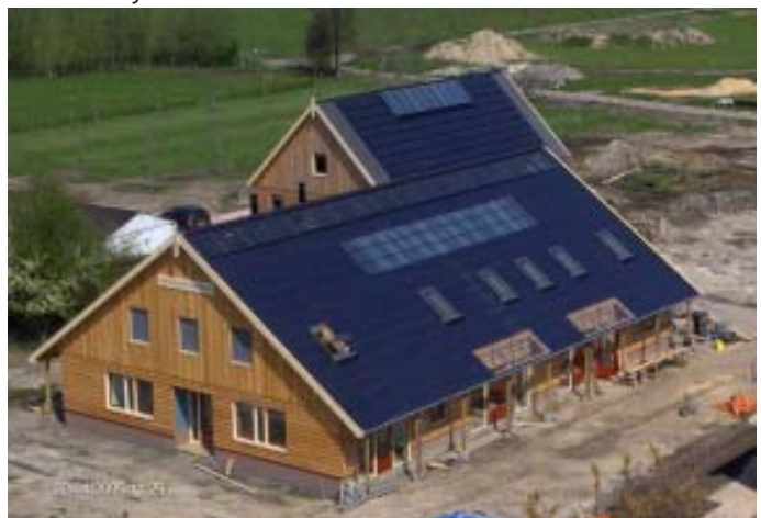
Black solar modules integrated into the roof of a new farm house in Netherlands.
